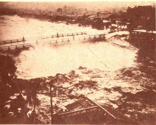
壞破淹被軌路車電快特神阪 The flooded Kobe-Osaka line.
