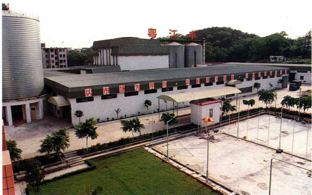
广州市江村家禽企业发展公司的江丰饲料厂 Jiangfeng Feed Factory of Guangzhou Jiangcun Chicken Breed Farm Company
