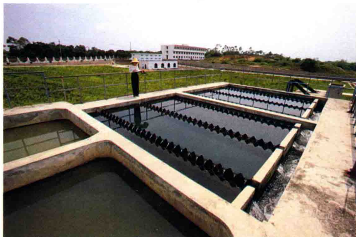
日产10万立方米的九佛自来水厂 Jiufu Water plant with 100,000 cubic meter water supply per day
