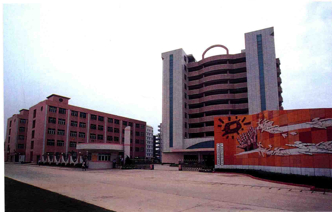
民办的广州白云职业培训学院教学大楼 The teaching building of Guangzhou Baiyun Vocational Training Institute run by the local people
