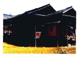
low ventilation at the same time, yaoyan is densely arranged with tiles, jutting out 1 to 1.5 meters from the walls, oblique with an angle of 25 to 30 degrees. This structure not only increases the stability of the construction, but also beautifies its appearance.
