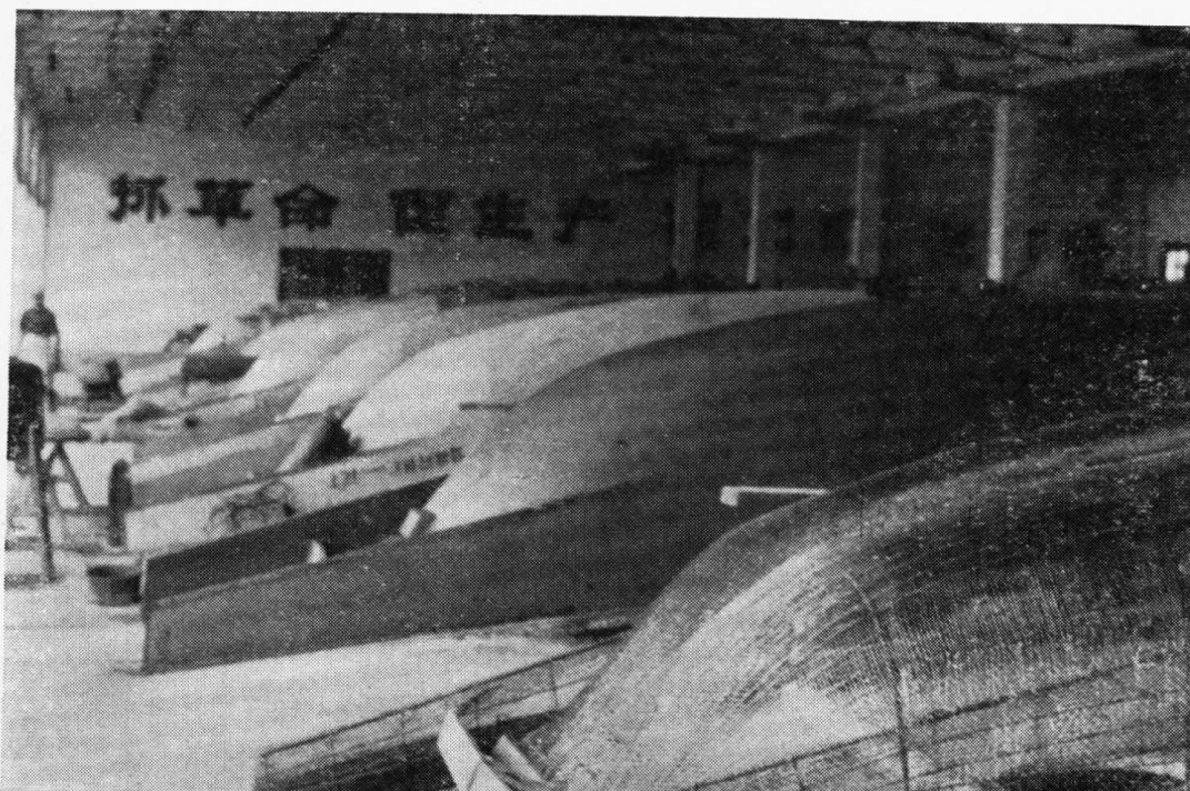
Concrete boats under construction in a Shanghai suburban commune.
