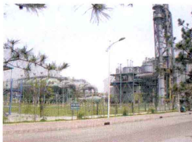
自主集成的转炉煤气干法除尘EP工程 Independent integrated converter gas dry-type de-duster of EP project
