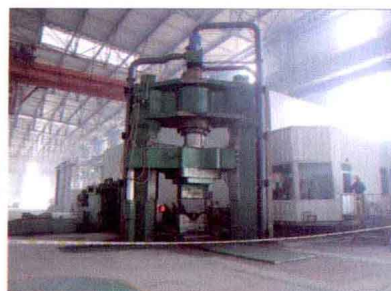
自主研发的20MN快速自由锻造液压机、80MN快速自由锻造液压机正在营口中试基地进行装配 Independent researched and developed 20MN fast free forging hydraulic machine, and 80MN fast free forging hydraulic machine is under installation in Yingkou pilot plant base
