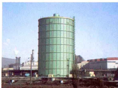
300000m 3 稀油密封圆型干式煤气柜 EPC总承包项目 300000m 3 Oil sealing round dry-type gas holder of EPC turnkey project
