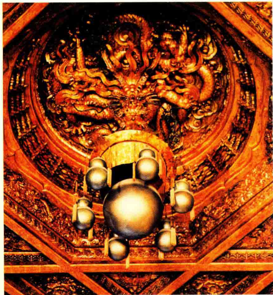
太和殿藻井 The Coffered Ceiling in the Hall of Supreme Harmony
