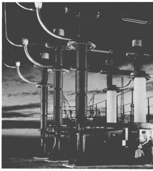
First 500,000 volt air-blast circuit breakers in U.S. commercial service. Evidence of industrial advances in the application of science. (Photo courtesy of General Electric.)
