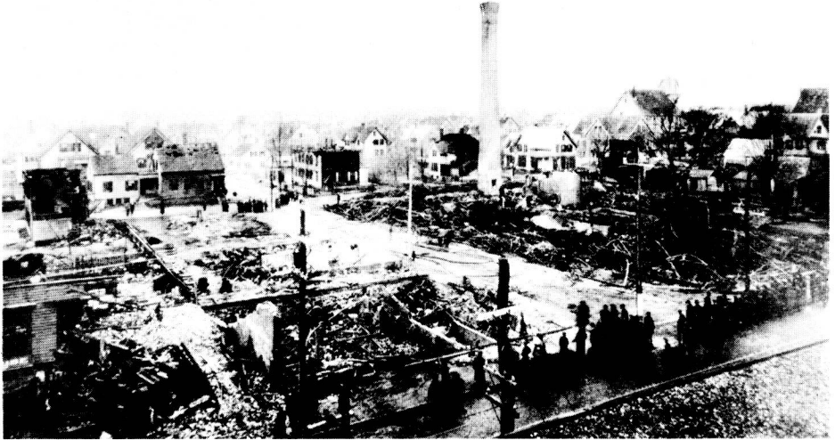
Figure 1.2 Shoe factory after the boiler explosion of March 20, 1905, which led to the adoption of many state boiler codes and the ASME Boiler and Pressure Vessel Code . (Courtesy of The Hartford Steam Boiler Inspection and Insurance Company .)
