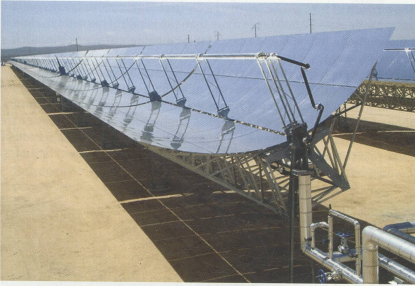
Figure 1.8: Solar thermal power station in California. The parabolic mirrors concentrate the sun's rays on the pipe to produce steam to generate electricity (Source: Solar Millennium AG, Erlangen, D)
