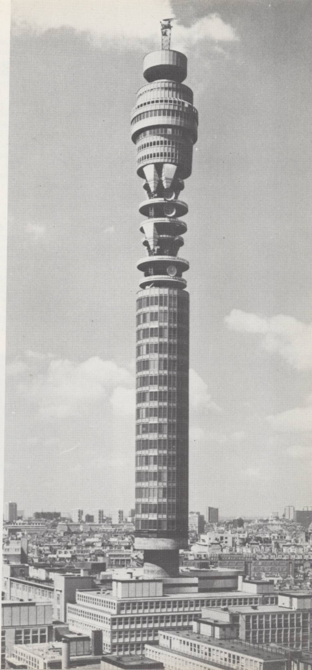
The Post Office Tower, London, showing the microwave antennae. By courtesy of the Post Office.
