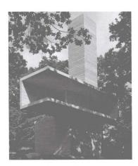
The 2008 pavilion for Kivik Art Centre in southeast Sweden, which has been designed by David Chipperfield and Antony Gormley, is open to the public until 28 September 2008. The pavilion, which was constructed in only two months, is a sculpture entirely in concrete. Formed of three interlocked 100 m³ volumes – 'The Cave', 'The Stage' and 'The Tower' – the pavilion offers three different ways of experiencing the nature and landscapes around Kivik.
