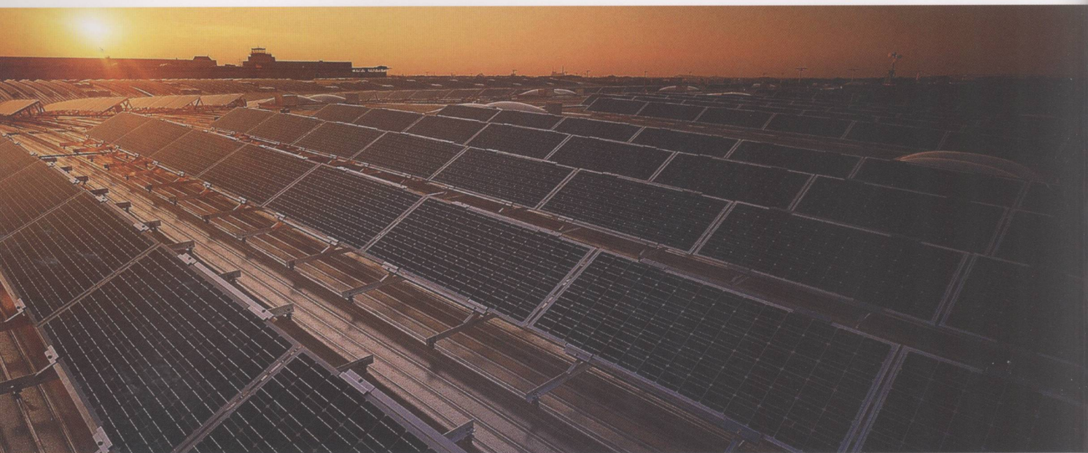
This large photovoltaic roof installation, above the Munich Fairgrounds building, has a nominal power output of about 1 MWe l. In 2004, it fed around 1000 MWh of electrical energy into the power grid (Photo: Shell Solar).
