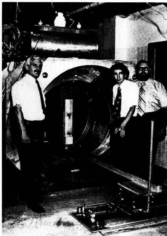
Figure 1-12. In 1977 Dr. Raymond Damadian and his associates, Dr. Larry Minkoff and Dr. Michael Goldsmith, successfully completed the construction of the world's first whole body MRI scanner. Named Indomitable to capture the spirit of its seven-year construction, it is now located at the Smithsonian Institute in Washington, D.C. (Courtesy Dr. Damadian and Fonar Corporation, Melville, New York.)
