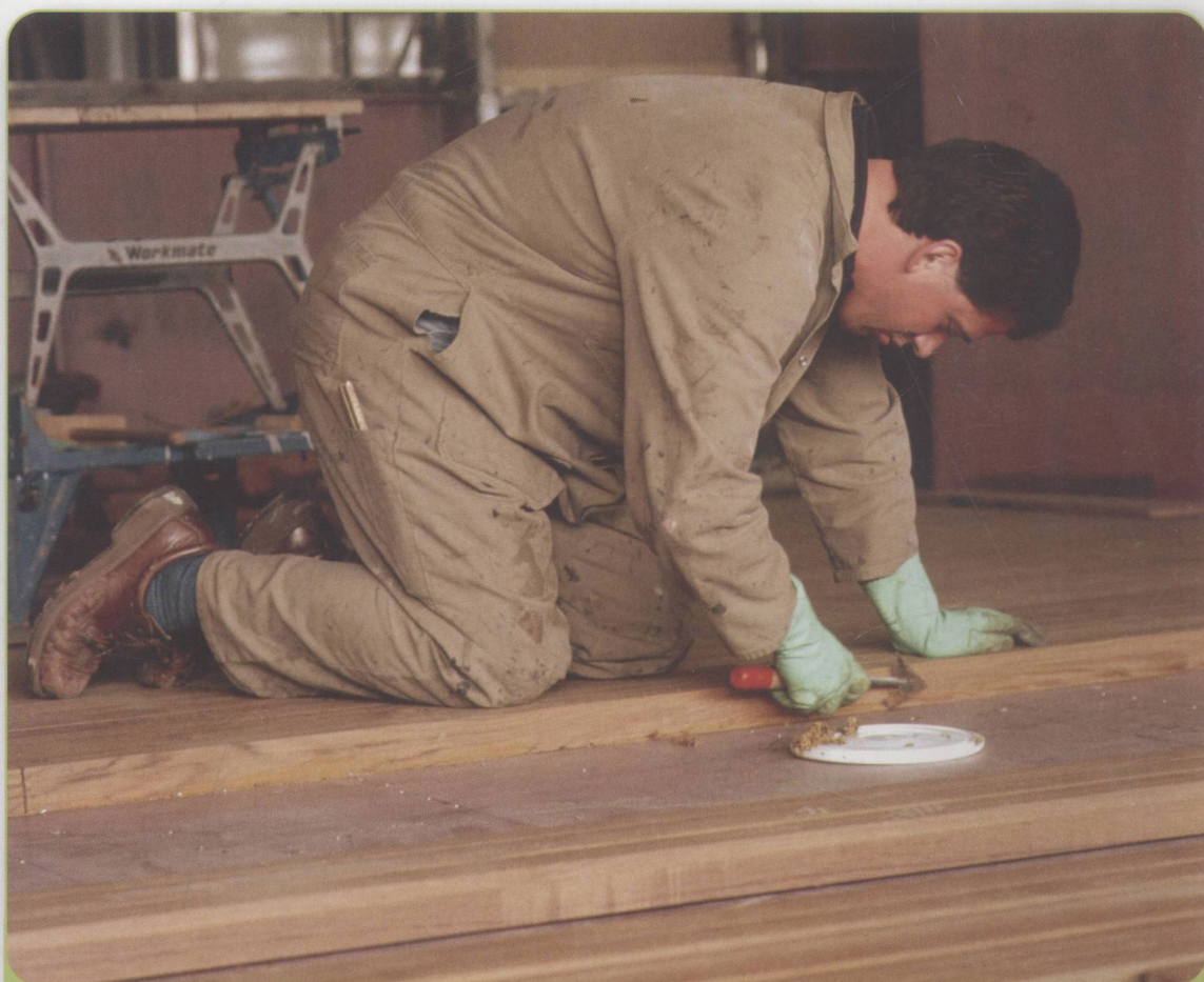
A carpenter lays teak decking on a ship.
