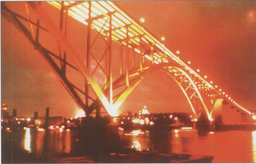
Figure 4 High Bridge over the Mississippi River, Minneapolis - St. Paul, USA, 1983
