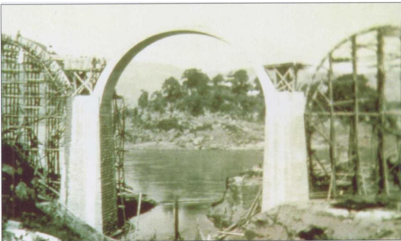
Figure 1 Three 20 m concrete arch spans, Cheng-Yu Railroad Bridge, China, 1938
