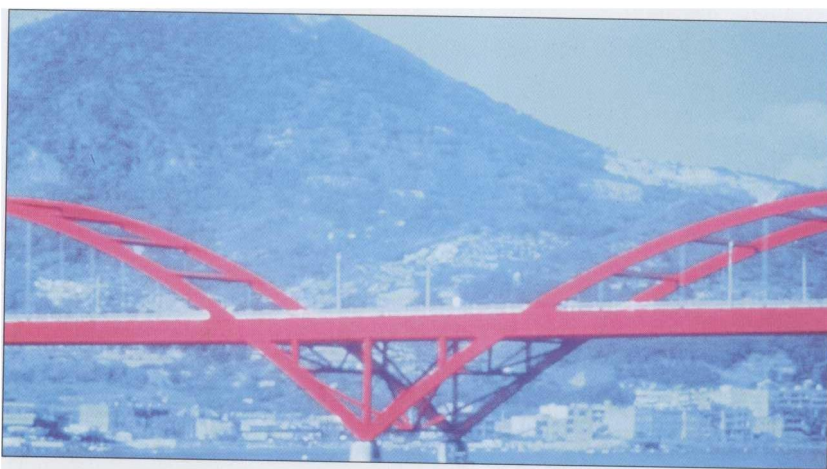
Figure 3 Kwang-Du Highway Bridge, Taipei, Taiwan, 1982
