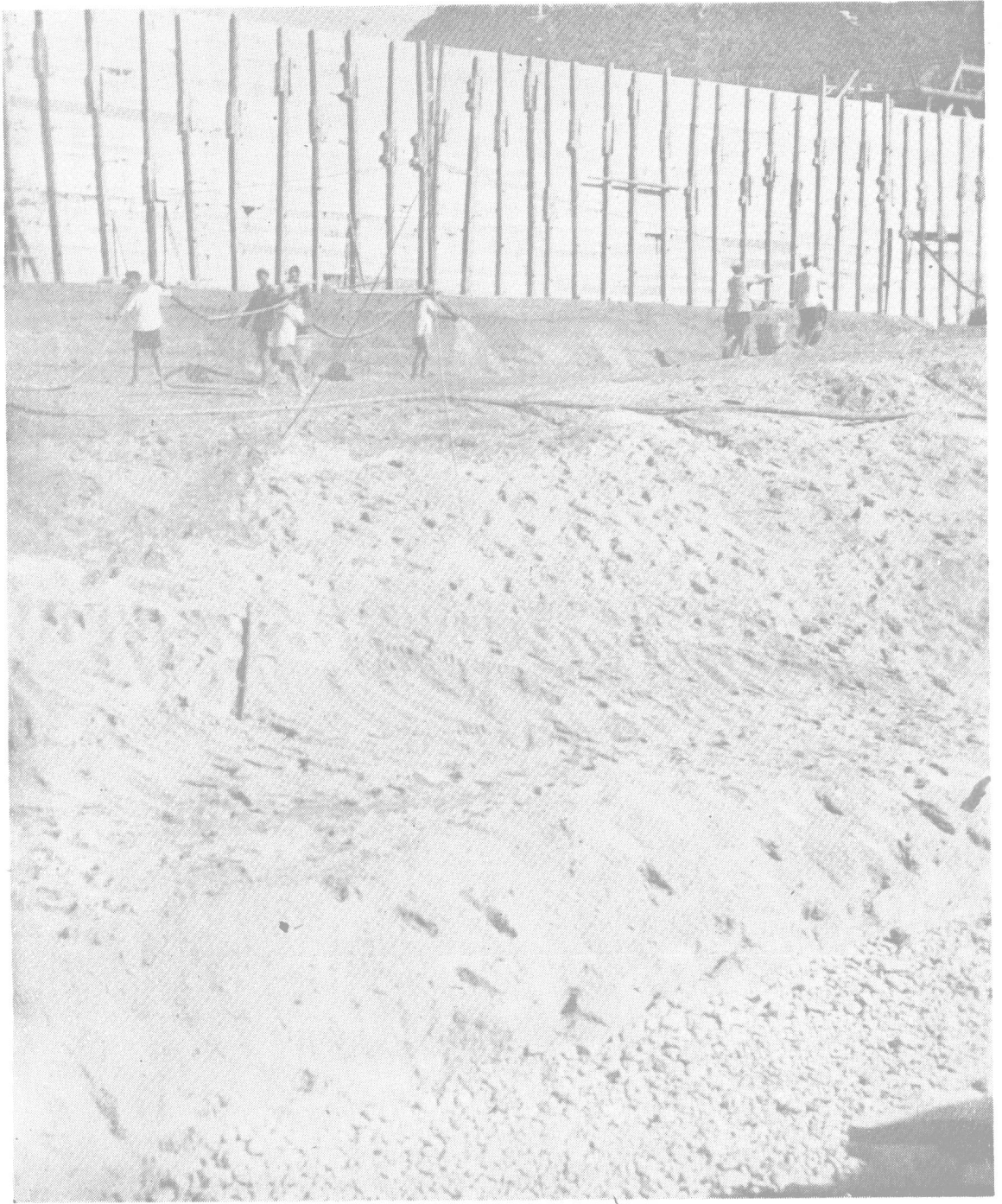
用“水冲填砂法”冲实木板心墙外砂壳
