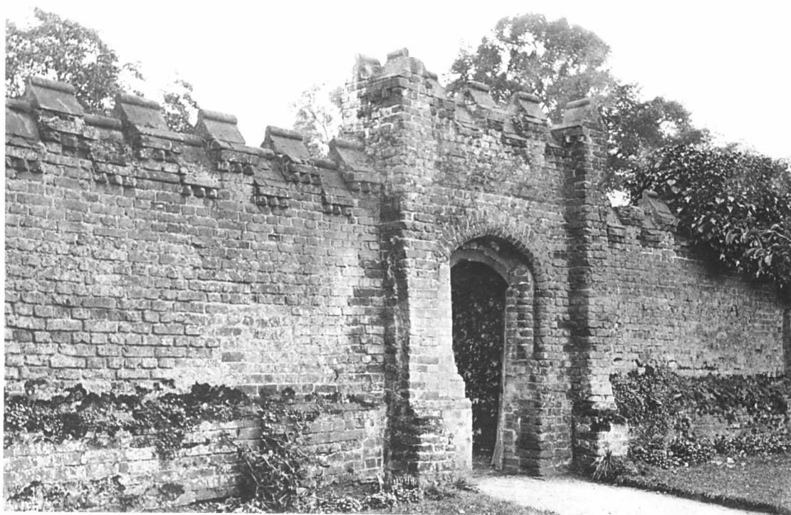
1-13 Breccles Hall, Norfolk. A notable example of the use of brick in the traditional Gothic manner. The design of the gateway is sufficiently massive to carry effectively its merely ornamental cresting of battlements.
