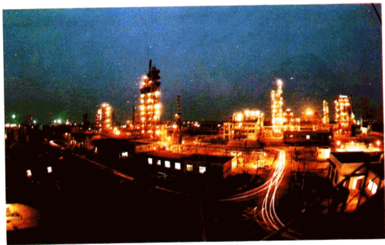
垦利炼油厂 Kenli Oil Refinery
