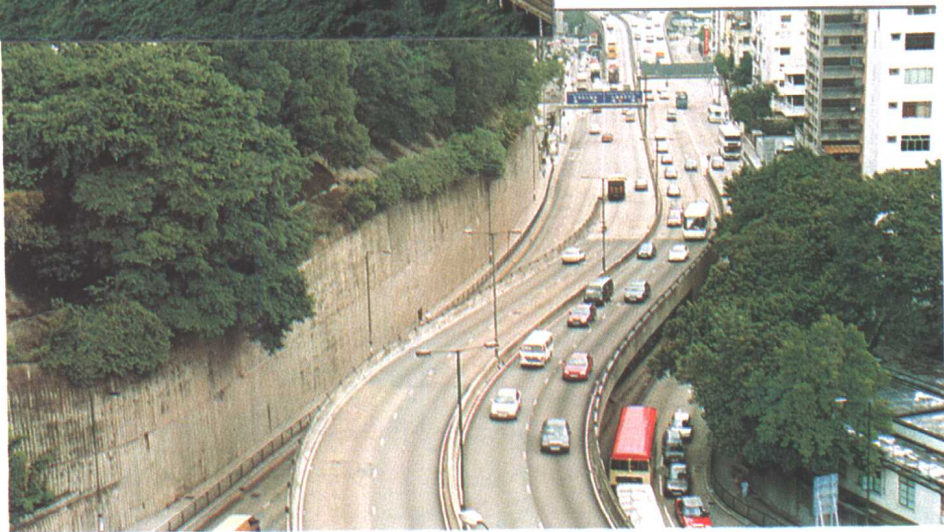
▶ 新公主道天桥, 1989年开通 (The new Princess Margaret Road Flyover)
