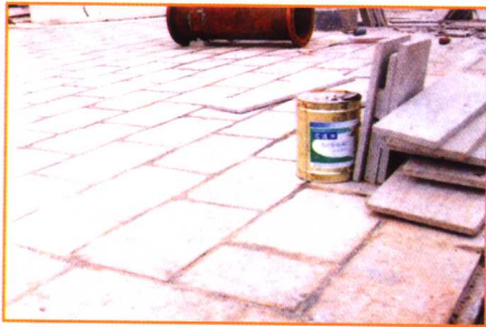
KPI胶泥砌筑花岗岩块， XLZ呋喃胶泥沟缝
