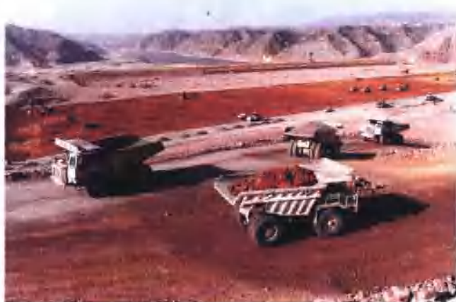
拦河大坝填筑
