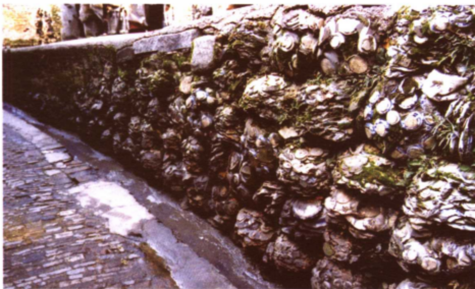
粘渣护坡 Dry slag protecting slope wall
