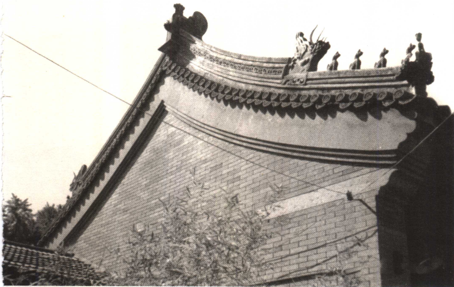
醇亲王北府东配房山墙
