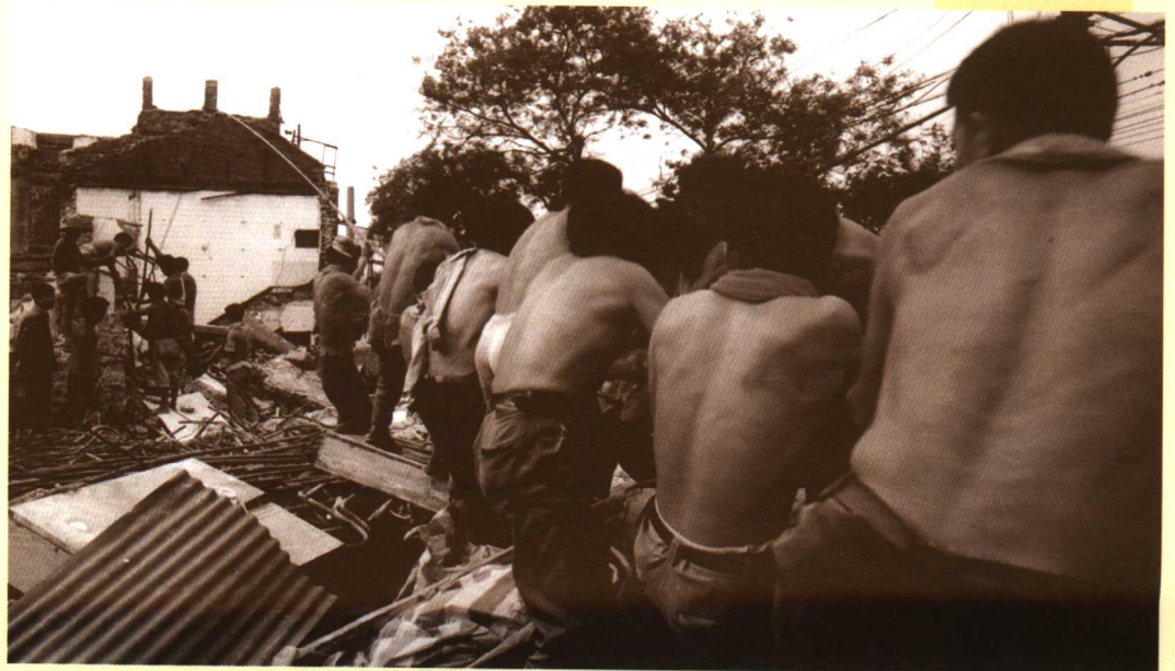
Jiefanglu Road under reconstruction
