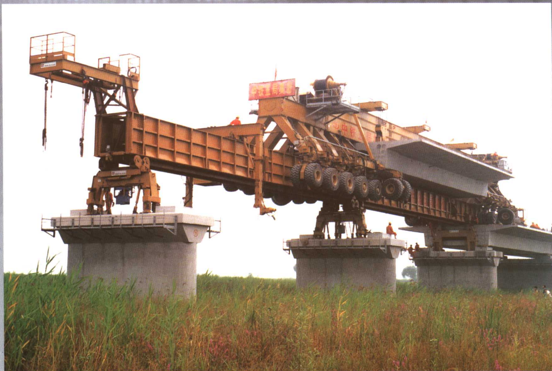
▲ 550t吊运架一体机运箱梁到达桥位，准备前移导梁
