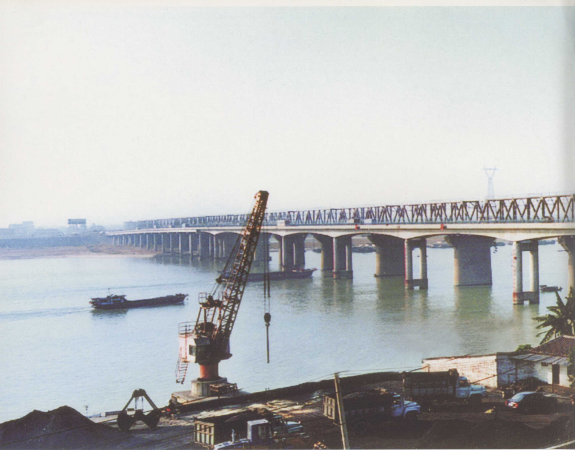
四会马房大桥 Mafang Bridge in Sihui
