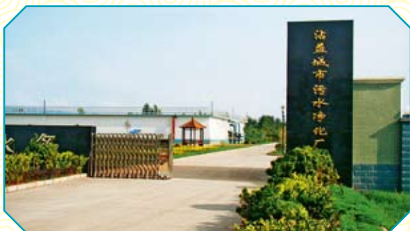
沾益城市污水净化厂
