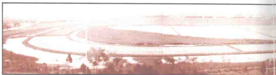
原汉口华商跑马场，现为学校体育场。 The former racecourse of Chinese businessmen, now the sports ground of the university.
