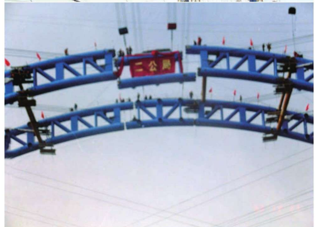
彩图30 190m跨拱肋安装合拢
