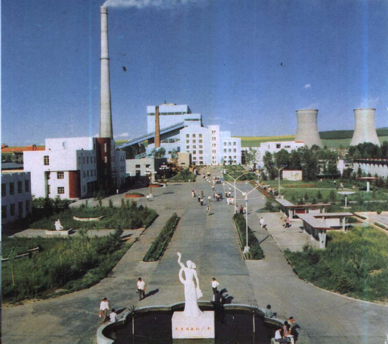
汇流河发电厂
