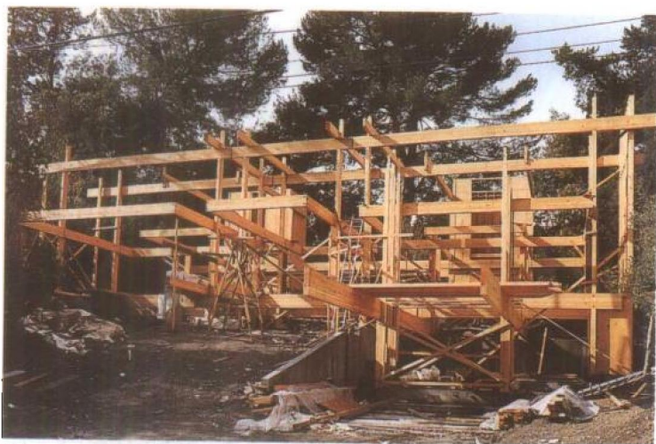
Katzenstein House, Pacific Palisades, 1973: (top) second-level gallery; (bottom) structural frame
