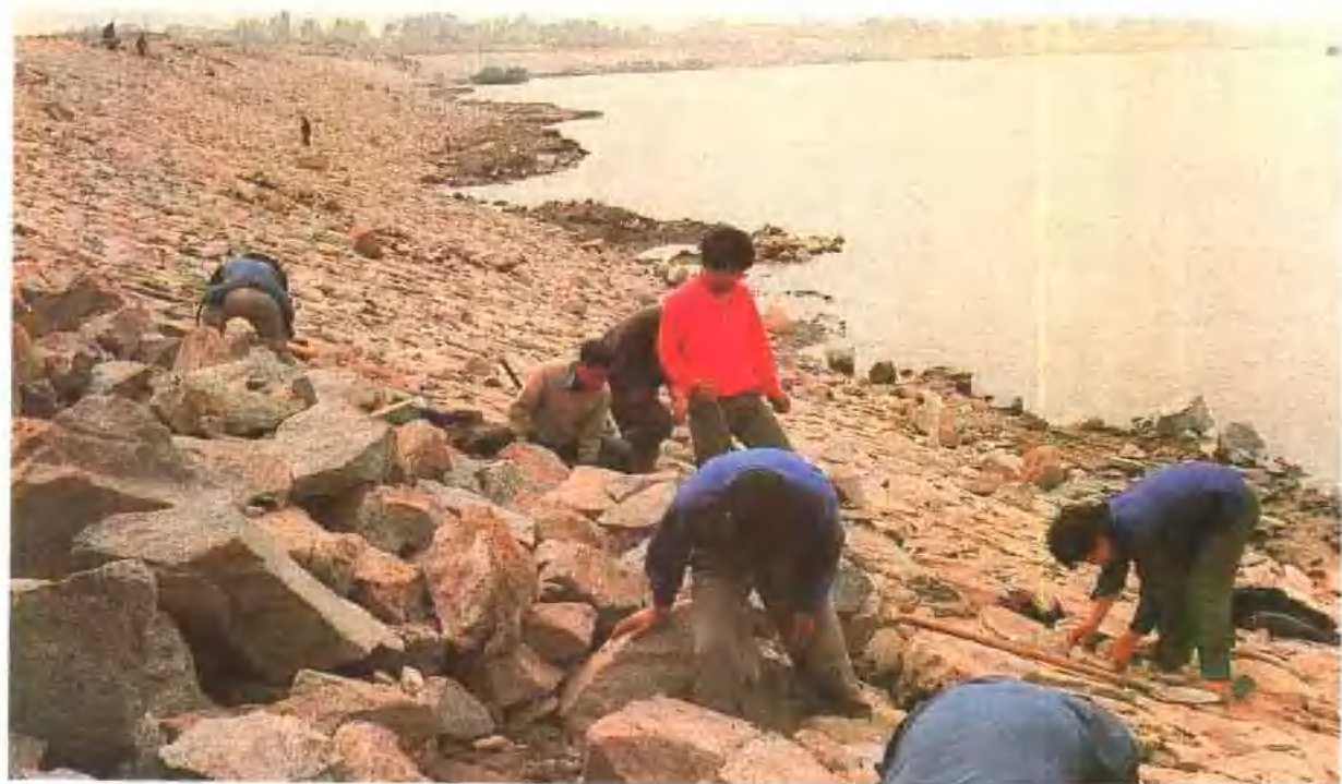
△块石砌坦护坡
