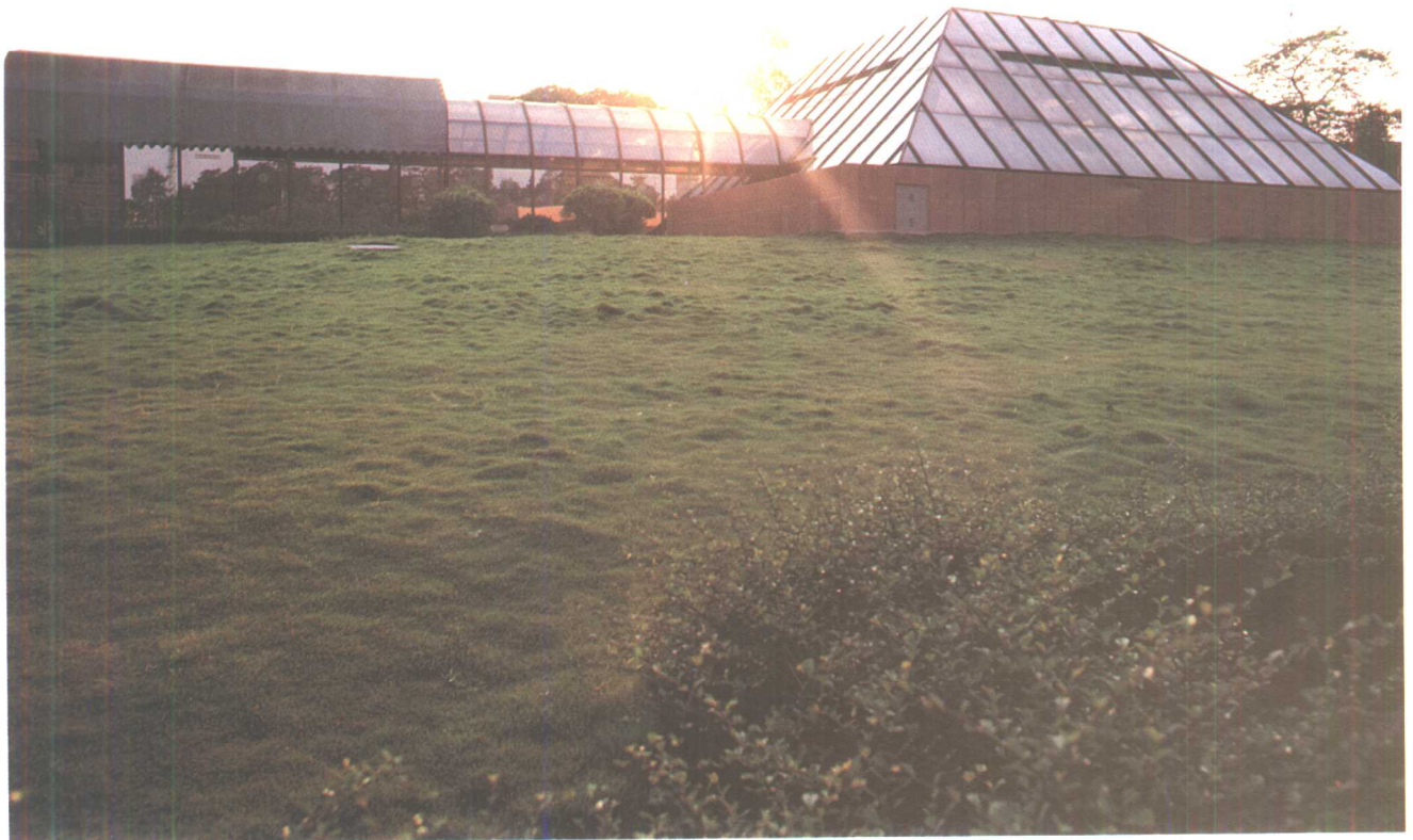
墓室修復後加建的玻璃棚保護罩外貌 Glass roof on top of the tomb chamber after restoration.
