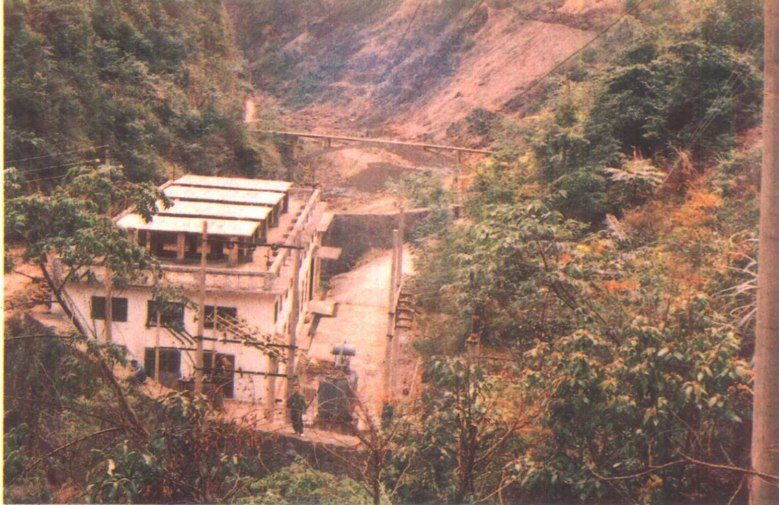
洞坎电站机房
