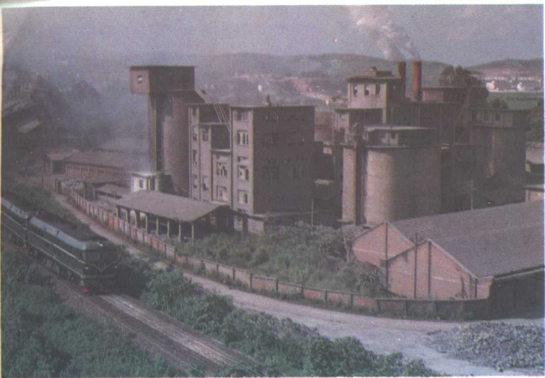
▲市水泥厂 ▶市合金电冶厂硅铁出炉 ▼市皮革厂
