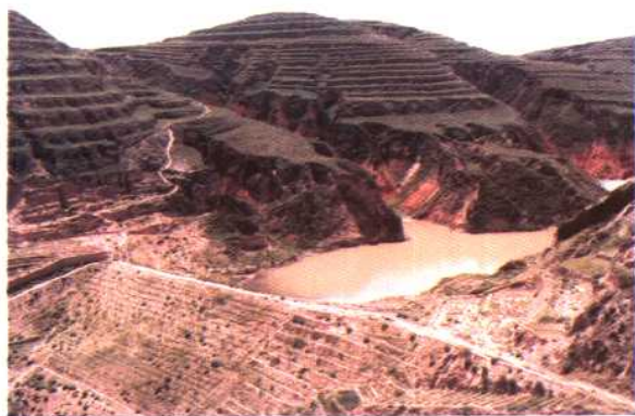
娄烦县凤凰沟淤地坝
