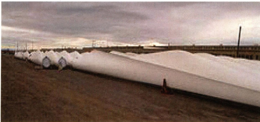
Fig. 1.1 Wind turbine blades awaiting installation in laydown yard
