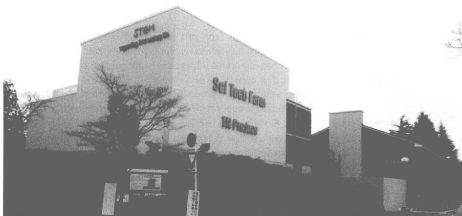
Fig. 1. Closed type commercial level plant factory in Tamagawa University.
