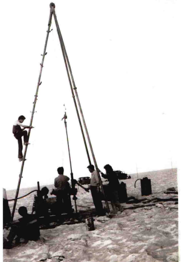
3-2 Building the drilling rig on the salt crust of Lop Nor
