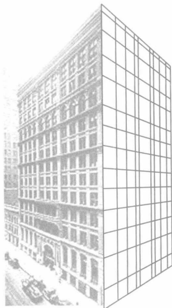
1884: Home Insurance Building, Chicago, William Le Baron Jenney. The 10-story structural frame of steel and cast iron carries the majority of the weight of the floors and exterior walls.
