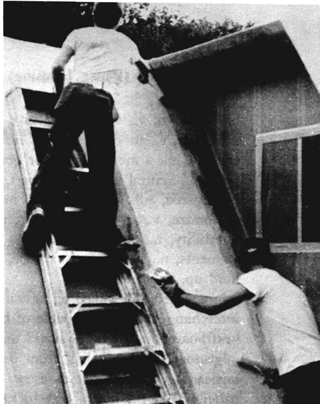
Picture No. 4: After the house has been erected, a coating of glass fiber and resin is applied to make it weatherproof. Source: Universal Papertech Corp.
