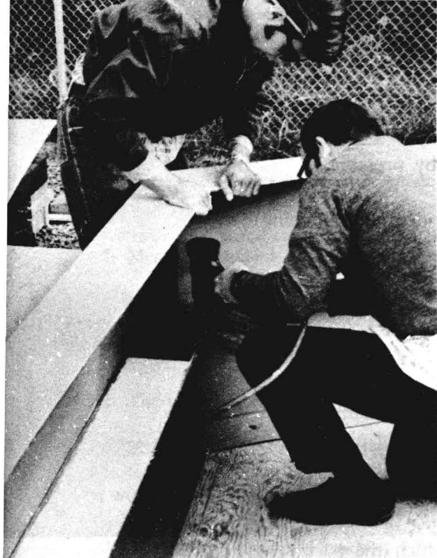
Picture No. 3: The sections of the houses are simply stapled together. Three workers can assemble a house in about 5 hours after the foundation has been built. Source: Universal Papertech Corp.
