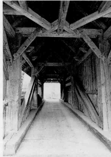
1 The joints of the diagonal bracing members on this bridge between Appenzell and Schlatt in Switzerland are so tightly restrained that settlement at the corner in the left foreground has caused the wood to split.
