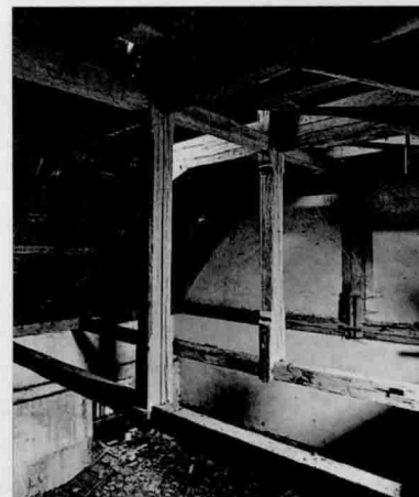
9 Two-part truss posts carry the tie beams in Schloß Thürntal, NE Austria.
