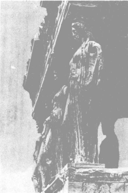
Fig. 6. Porch of Maidens of the Erechtheum on the Acropolis in Athens, showing the effects of air pollution on the statues
