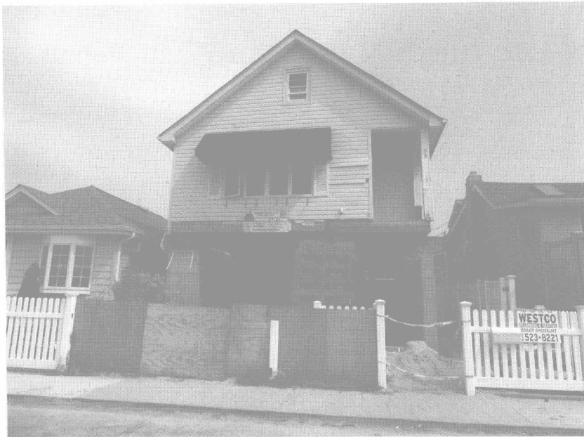
Figure 1.1 This home was damaged in Superstorm Sandy and is in the process of being lifted up to avoid future damage. Damage from hurricanes is increasing around the world.
