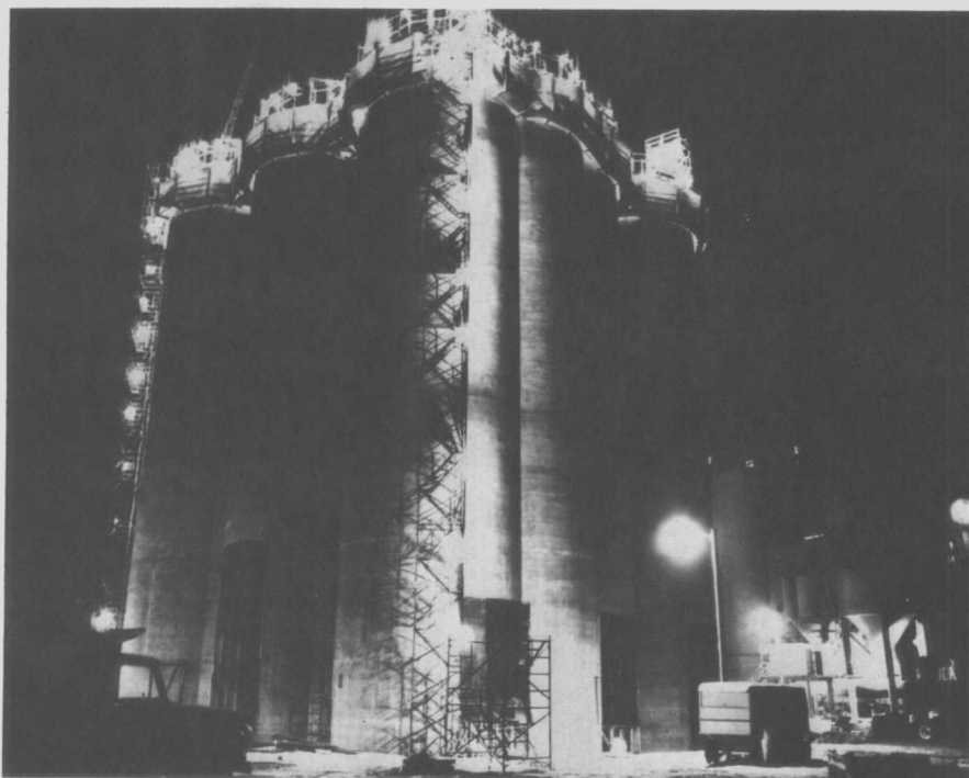
Plate 1-1. Around-the-clock slipforming of cement storage silos at Portland, Colorado. (Courtesy of Ideal Cement Co.)
