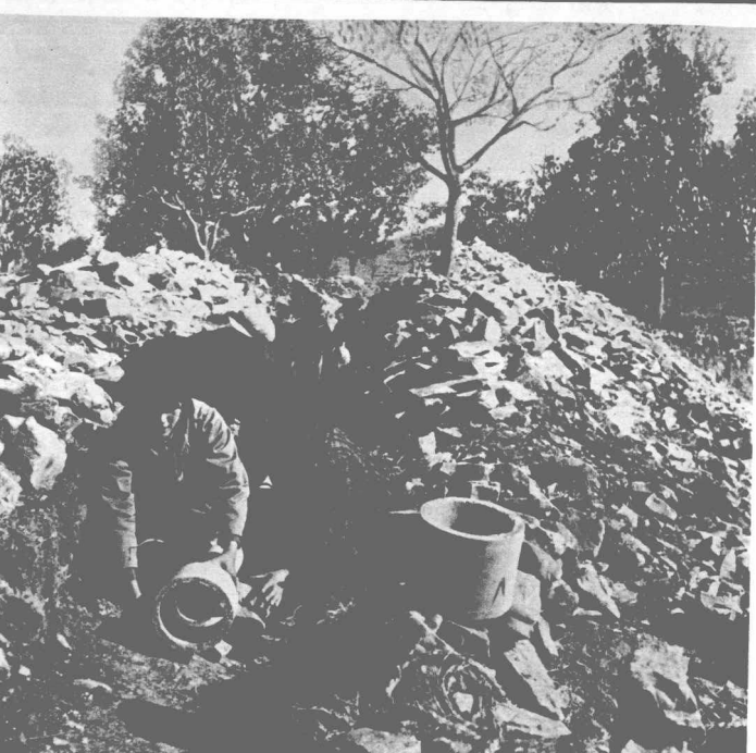
Laying a pipe- line to conduct the water.
