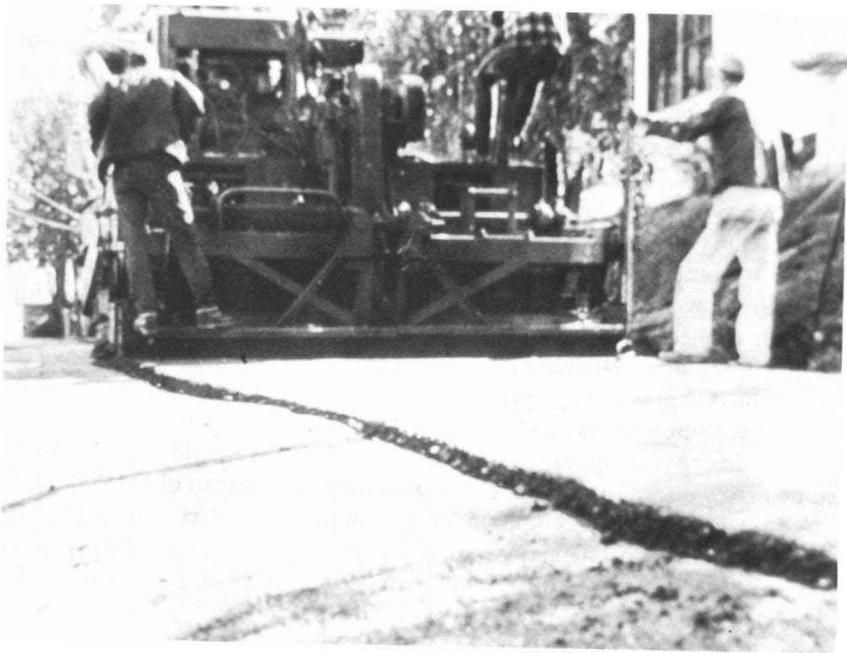
FIG. 5—The leveling action of the floating screed.
