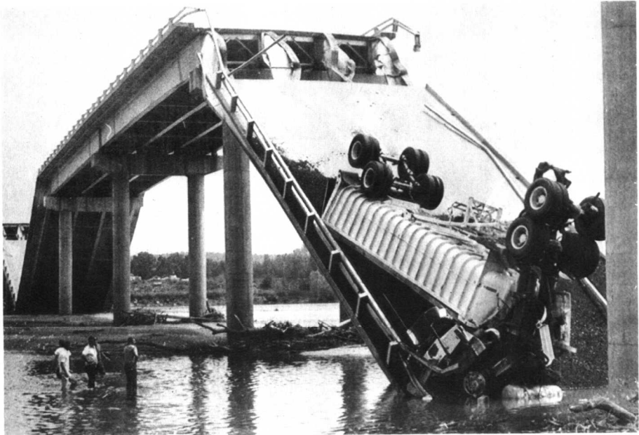
Figure 1-1 The South Canadian River Bridge on U.S. 75 near Calvin, Oklahoma, fell on May 21, 1976. Drivers of two semitrailer trucks were killed. The expansion joints at each pier apparently locked, so that all expansion and contraction accumulated at one joint. When the span “walked” off the pier at that point, it dragged other spans with it. ( United Press International. )
