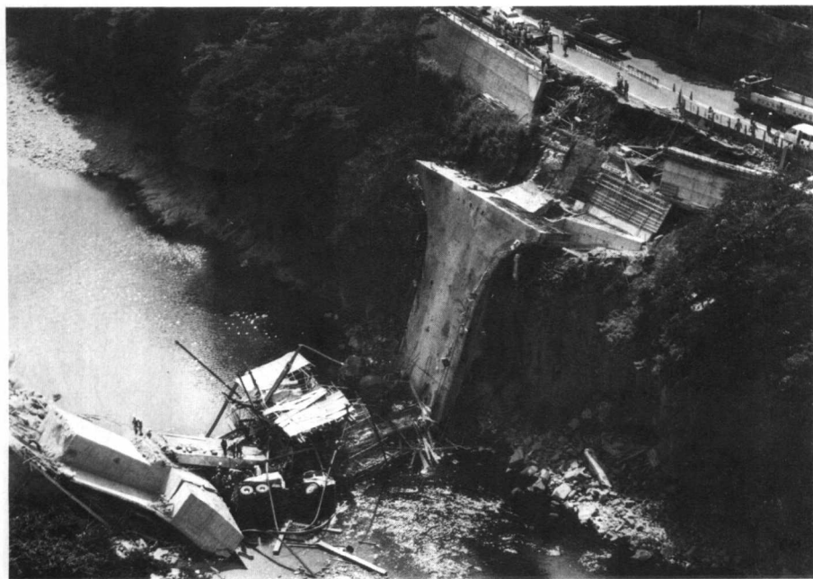
Figure 1-7 Formwork failures are among the most common of all construction disasters; formwork design is often left to nonprofessionals. This collapse occurred in Japan in 1978. (Kyodo.)
