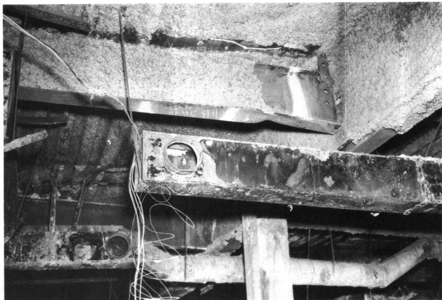
Figure 1-6 Modern construction can be remarkably immune to fire—although loss of life and damage to interior furnishings can be substantial. Here, the basic soundness of framing at 1 New York Plaza is evident after a 1970 blaze. ( Alfred H. Miller Co. )
