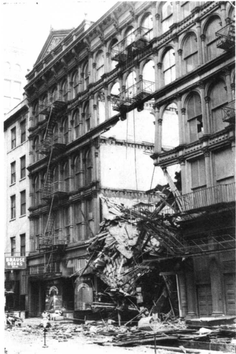
Figure 1-2 This overloaded loft building on Duane Street in New York City collapsed late in 1944. The facade was mass-produced cast iron, made to look like stone, which was popular in New York before the turn of the century. ( ENR File. )
