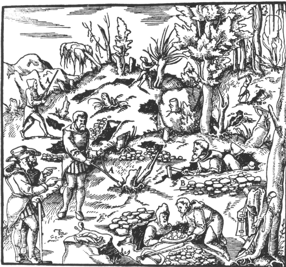
FIG. 1.1. Prospecting with a forked stick (A) and trenching (B) in the fifteenth century (from: Agricola, De Re Metallica , translated into English, Dover Publications, New York, N.Y.).
