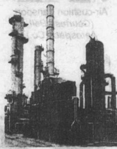
Alkylation section of a refinery (Courtesy Econo-Therm Corp.)
